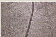
Cleaned crack
