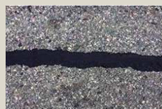
Sealed Crack
